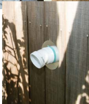
Figure 4. A plumber installs a section of flue pipe (above left), taking care to slope it so that condensate drains back to the heater. With the particular heater shown here, the flue can be ABS or PVC; in this case, it's a combination of the two (above) because the plumbers ran out of ABS. The flue passes out through the wall and terminates at a screened fitting (left).
