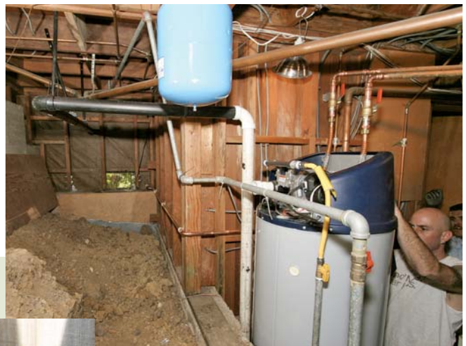
Figure 4. A plumber installs a section of flue pipe (above left), taking care to slope it so that condensate drains back to the heater. With the particular heater shown here, the flue can be ABS or PVC; in this case, it's a combination of the two (above) because the plumbers ran out of ABS. The flue passes out through the wall and terminates at a screened fitting (left).
